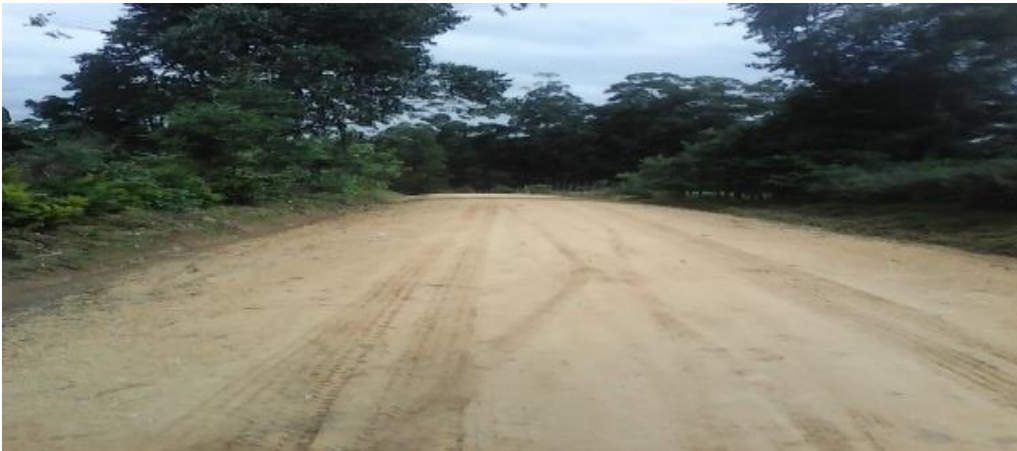
SECTION OF MUDUNGU-NABWANI ROAD
