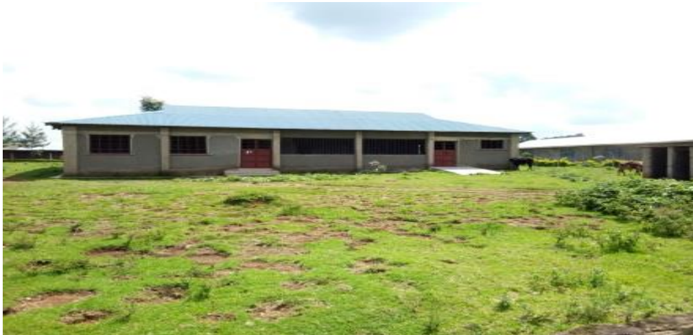
SHIPALA DISPENSARY UNDER CONSTRUCTION
